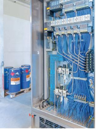
The new solution greatly reduces the space and installation work required, because only the electricity supply and Profibus cable need to be connected.
