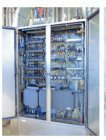
The size of the valves in the old Bürkert cabinets meant that only a limited number of pneumatic signals were possible. The "EX-e" wiring was also a great deal more complicated.
